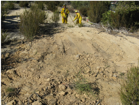
Photo 7: Prior to commencement of soil test pit excavations, an environmental monitor is required to instruct crews on the methods to salvaging the topsoil onsite. Fire crews were observed conducting fire prevention activities at the test pits post- excavation.
