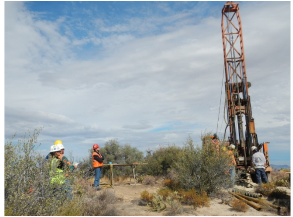
Photo 6: Biological, archaeological, Native American, and fire monitors observe a drill rig used for geotechnical boring/drilling activities. Temporary work space measuring approximately 40 x 60 feet is utilized to complete geotechnical testing activities at each testing location.
